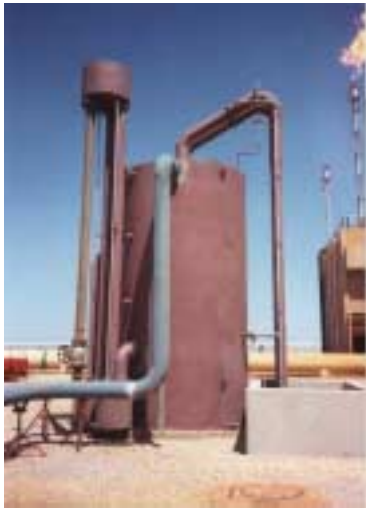
Chemical Industry South Africa Side-Stream Filtration of Cooling Water Circuit 1 Double Bed Flow 200 m 3 /hr
