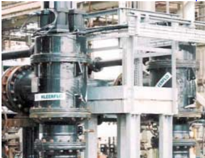
Chemical Industry UK Duty/Standby 1400 m 3 /hr each Sea Water Cooling
